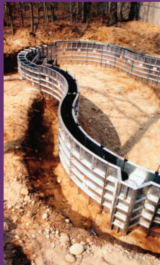
Aluminum forming systems can be used to create concrete wall vinyl-liner pools in virtually any shape.
