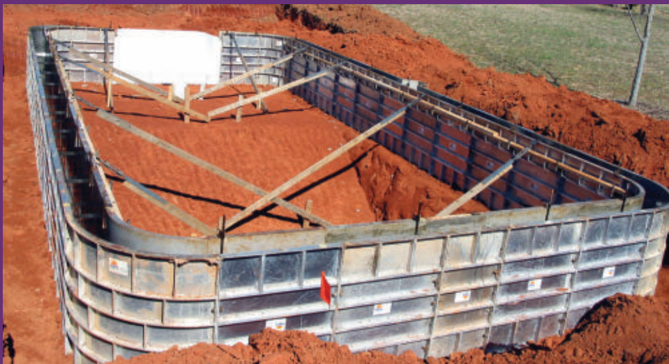
Some pool builders are purchasing their own aluminum concrete forms to control costs and avoid the long wait for materials like steel.
